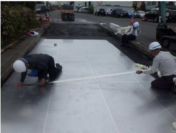
(a) Perforated metal (GND) on the ground
