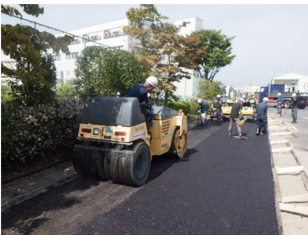
(c) Bituminous stabilized material on the drainage course
