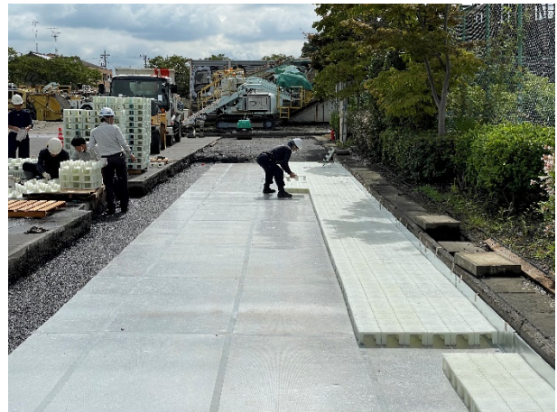
(b) Drainage course (Reinforced Plastic) on the GND
