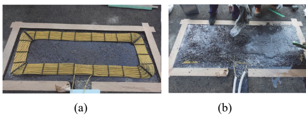
Fig.6 Coil 10 buried with resin, (a) coil installation after drying of MMA resin, (b) MMA resin + silica sand
