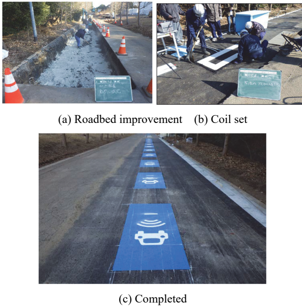
Fig.5 Pictures of coil burial work
